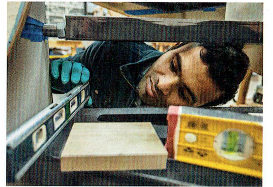
Ayad takes precise measurements for the placement of a stair tread while building a staircase. Katzoff says NK Woodworking & Design "really transitioned to a legit company" over the last few years. "What really got the national attention is our design ability — that's my best skill, as creative director and designer."
